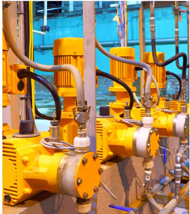
However, VFDs come with a consequence: they create an electrical discharge that causes premature pitting and motor failure. Having to replace a motor years early can quickly cut into electric savings. EGS therefore performs electrostatic testing to identify the problem, then installs shorting rings to give the electricity a non-damaging path out of the motor.
